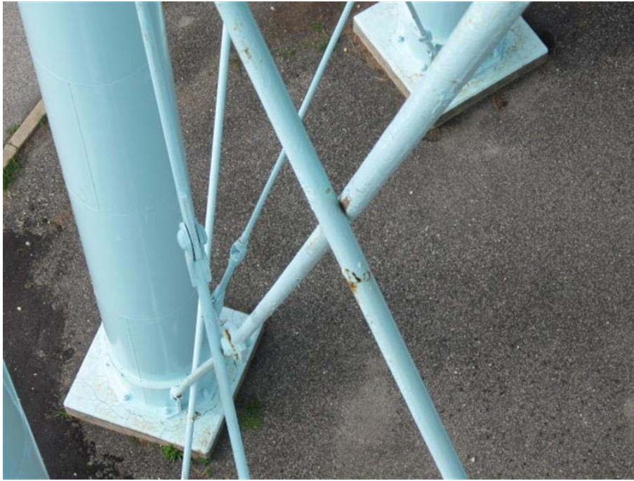
Photo #35 Wind rods are tight and in good condition.
