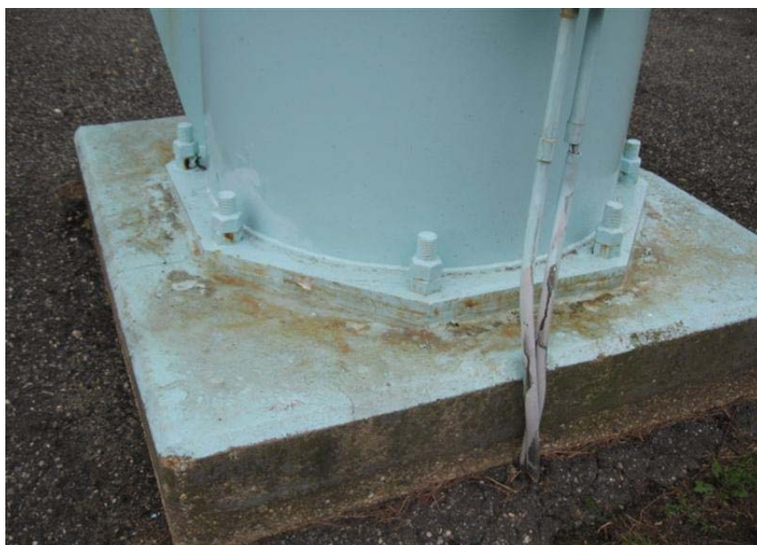
Photo #39 Approximately 6 anchor bolts and nuts exhibit severe levels of corrosion and should be replaced during the next renovation.
