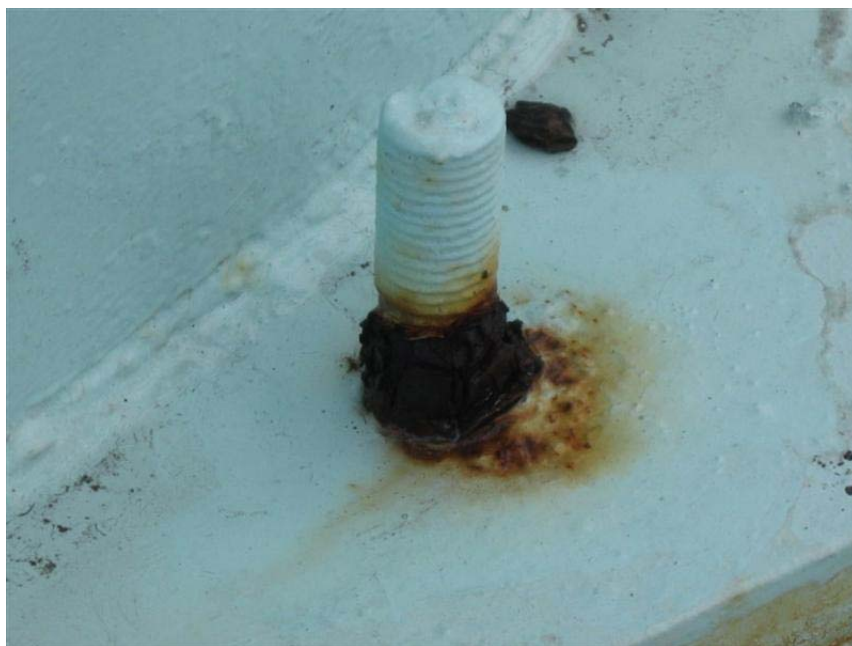
Photo #39 Approximately 6 anchor bolts and nuts exhibit severe levels of corrosion and should be replaced during the next renovation.
