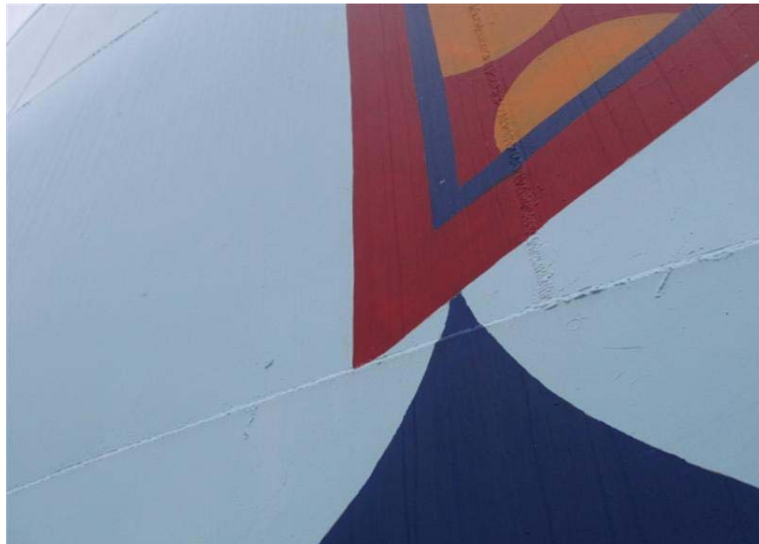
Photo #10 Coatings on sidewall are in good condition
